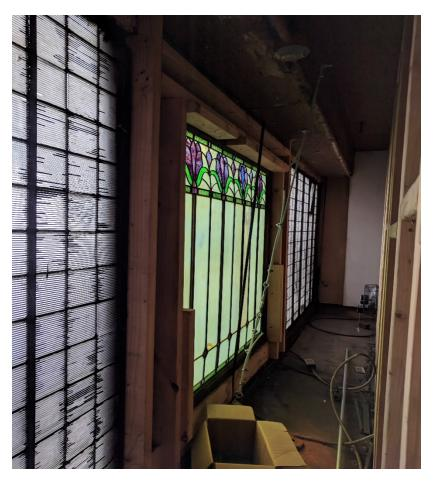
The reason for the change per the tenants was too much structural damage...this is a picture from behind of how the framed the new stained glass to be removed. We will keep the framing but on the exterior limit the visible framing to 1 inch.
